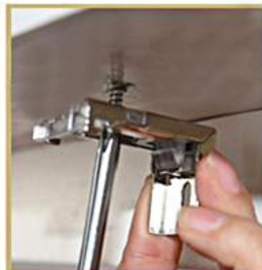
04. Fix the mounting hardware into the wall
